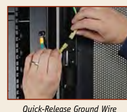
Quick-Release Ground Wire
