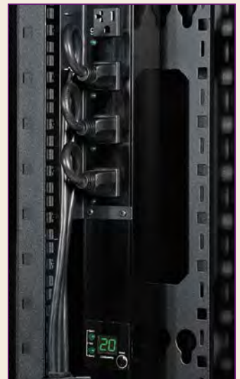
Toolless installation of a Tripp Lite PDU—simply insert the mounting buttons into the mounting slots and slide downward.
