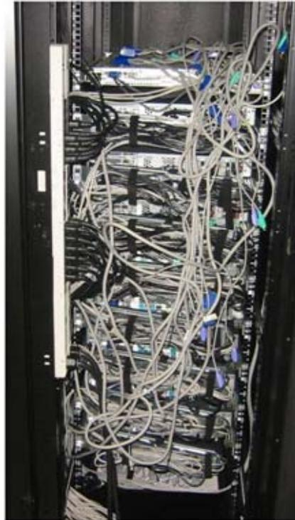
**Figure 4. Poor in-cabinet cable management practices introduce clutter and choke points in the exhaust area that limit cooling system effectiveness.**
