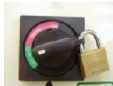
(a) Lockout for Energy Isolating Device
