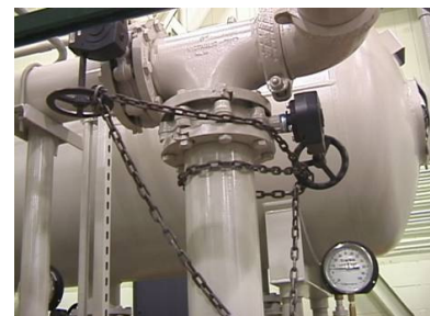
(b) Lockout for Hydraulic Valve
