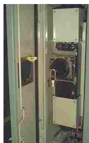
(a) Lockout for Energy Isolating Device
