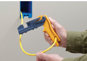
1. Strip cable jacket with a standard cable stripper or the built-in cable stripper.
