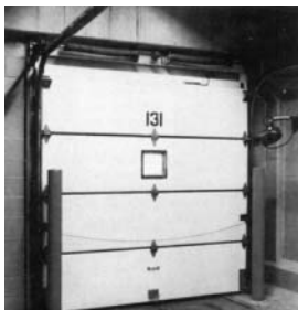
Limit Switches Help Operate This High-Speed Door
